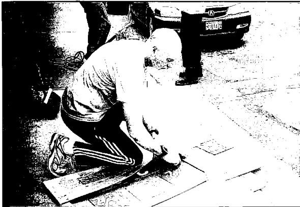
Dr. Hogan unwrapping the "green" mile markers just installed on the Gig Harbor waterfront route
